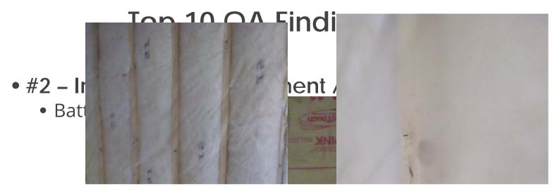
2. "Grade II" shall be used to describe an installation with moderate to frequent installation defects: gaps around wiring, electrical outlets, plumbing and other intrusions; rounded edges or "shoulders"; or incomplete fill amounting to less than 10% of the area with 70% or more of the intended thickness (i.e., 30% compressed); or gaps and spaces
